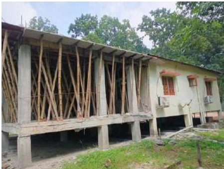
Extension of Director Residence under progress
