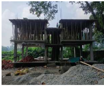
Construction of two storied staff quarter under progress
