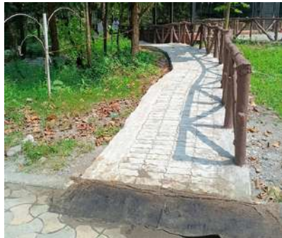
Construction of visitor footpath in the snake house section
