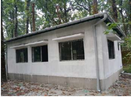
Construction of guest house under progress
