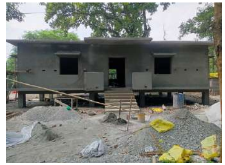
Construction of Assistant Director residence under progress
